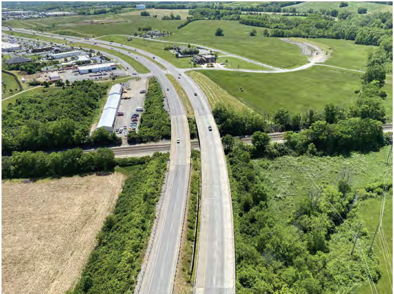
View of Danville Bypass
