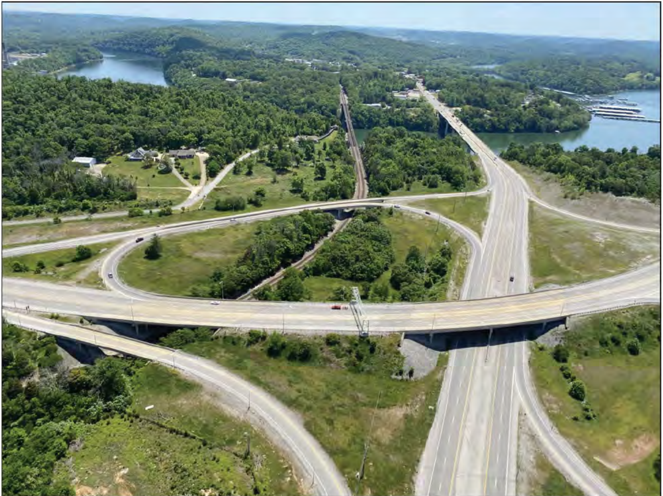
View of the line headed south at the Cumberland River, Burnside, Pulaski County, KY
